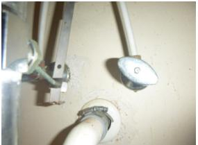
3. ALL THREE BATHTUB VALVES LEAK WHEN ON. APPROXIMATE REPAIR COST. \$45 - \$95 EACH
