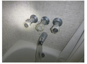
4. BATHTUB SPOUT IS CORRODED WITH SHARP EDGES. APPROXIMATE SPOUT REPLACEMENT COST. \$45-\$65
