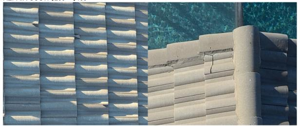
THE ROOF IS SLOPED WITH AN "S" TILE OVER MEMBRANE ROOF SYSTEM. THE ROOF IS THE ORIGINAL, APPROXIMATELY 17 YEARS OLD. THE ROOF IS IN SATISFACTORY CONDITION AND CURRENTLY LEAK FREE. THE NORMAL MAXIMUM ROOF LIFE, FOR THIS TYPE OF ROOF SYSTEMS 25 YEARS.
