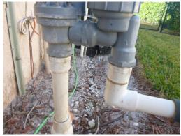
3. THE INDEXING VALVE IS STICKING, CONSEQUENTLY IT IS NOT CHANGING ZONES PROPERLY. APPROXIMATE REPAIR COST. \$150 – \$300
