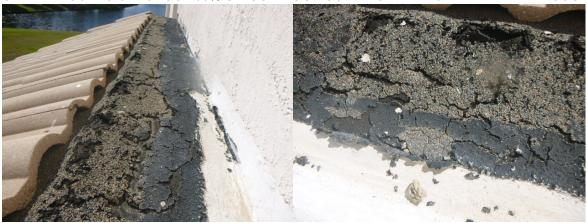
2. THERE IS APPROXIMATELY THREE DOZEN SMALL CRACKED CORNERS OF ROOF TILES. THERE IS ONE TILE AT THE SOUTH END THAT IS CRACKED FULLY THROUGH. ALL DAMAGED TILES SHOULD BE REPAIRED WITH THE APPROPRIATE ROOF ADHESIVE, SUCH AS RT 600 OR POLY FOAM. APPROXIMATE REPAIR COST. \$200 – \$400
